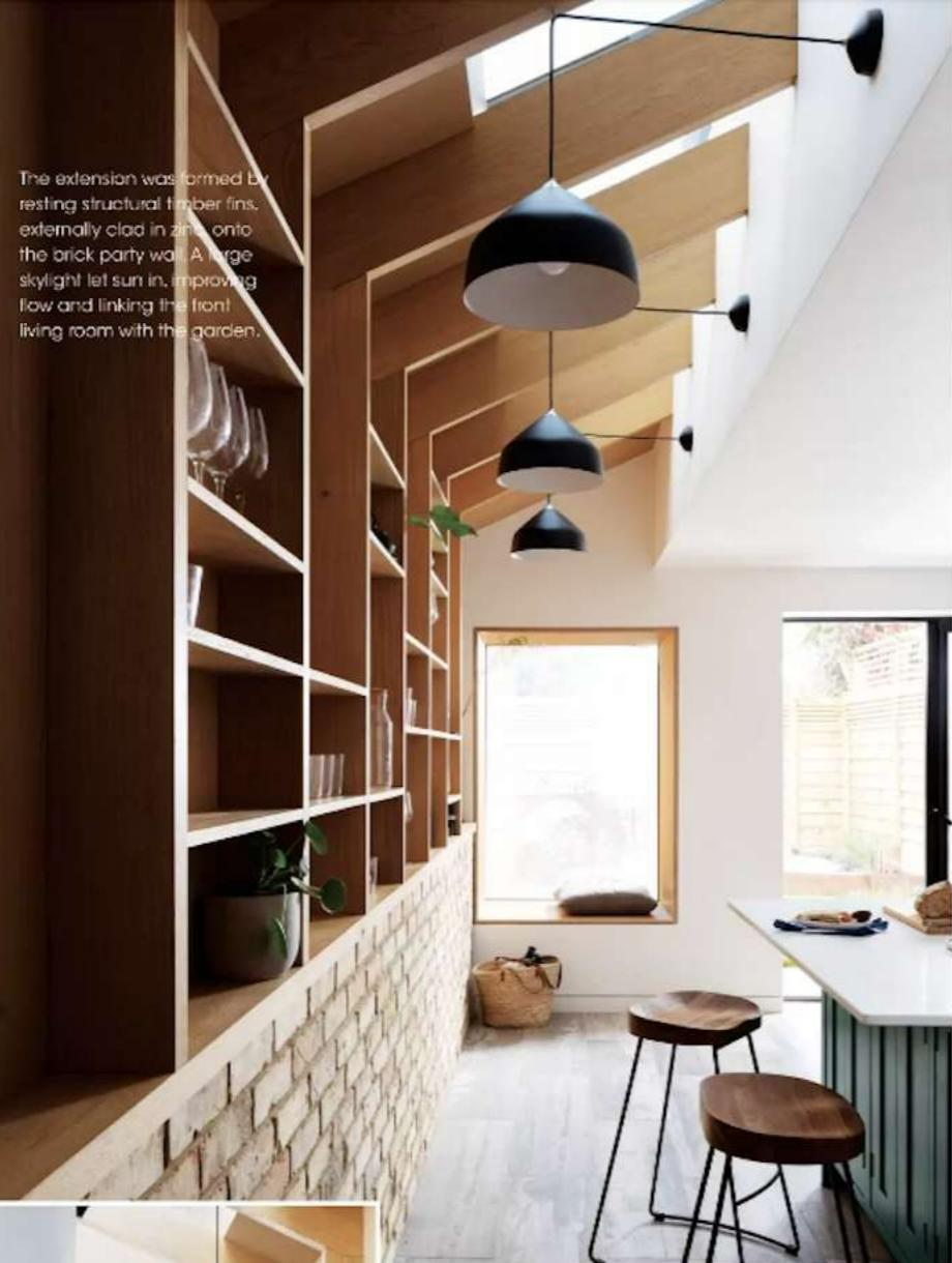
The extension was formed by resting structural timber fins, externally clad in zinc, onto the brick party wall. A large skylight lets sun in, improving flow and linking the front living room with the garden.
